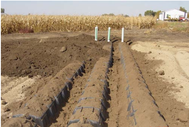
At Grade Subsurface Sewage Treatment System
